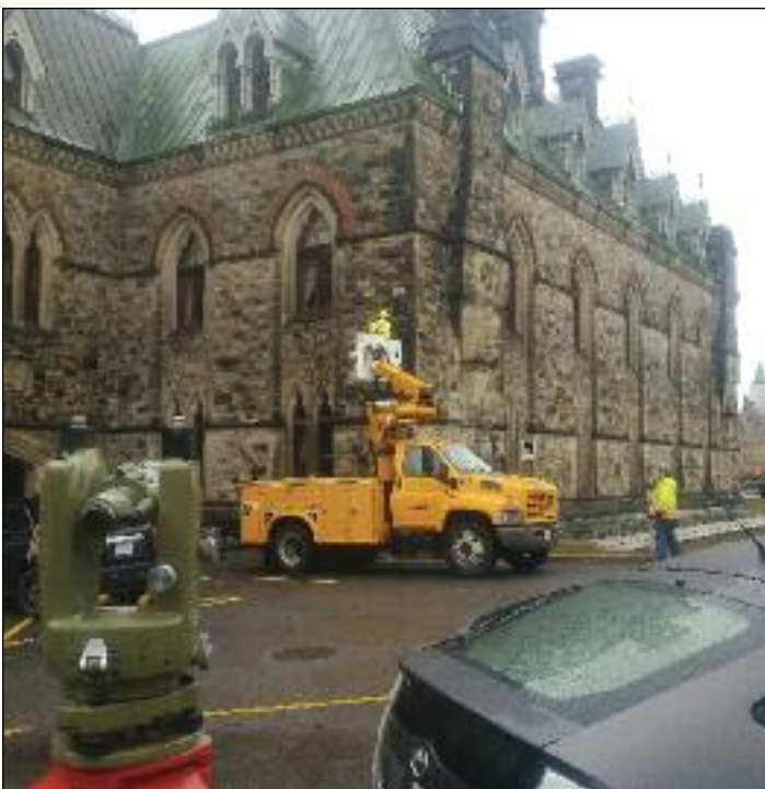
Figure 2: Installation of wall-mounted prisms on one of the East Block's facades by employees from PSPC. The prisms were aligned by the FMW surveying team using a theodolite.
