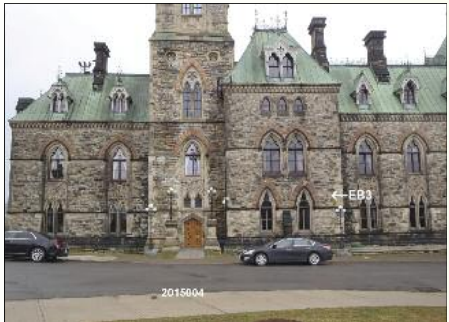
Figure 1: The control network is made up of monuments on the ground and prisms mounted on the walls of the buildings. Here, there are two points near the East Block. Some points, including 2015004, were installed to connect the existing interior networks of the Parliament Buildings to the new geodetic network.
